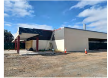
400 Building Water barrier and stucco
